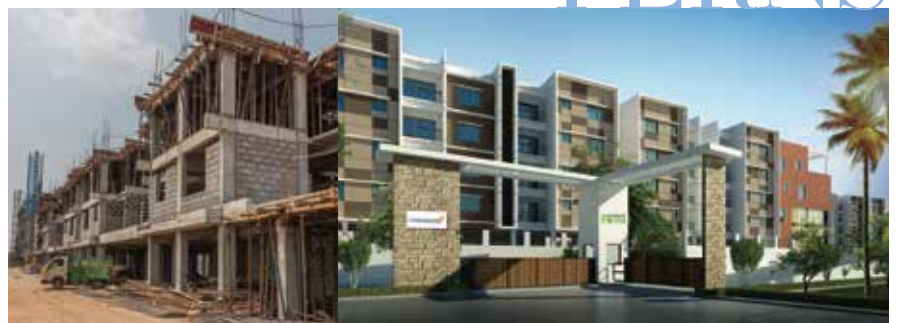
Casagrand Ferns @ Tambaram • Roof slab work in progress
