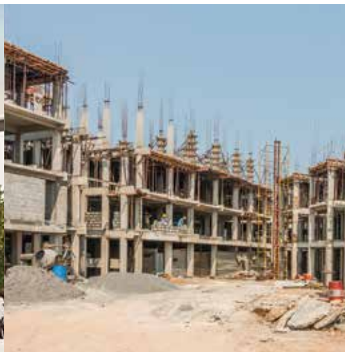
Casagrand Bellissimo @ Alandur • Roof slab work in progress
