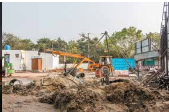
Casagrand Olympus @ Mandaveli • Foundation work in progress
