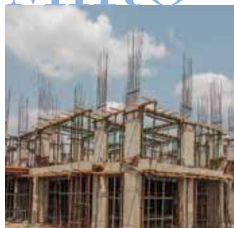
Casagrand Miro @ Mannivakkam • Roof slab work in progress
