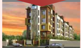
Casa Grande Lanterns Court Residential Apartments, Thoraipakkam
