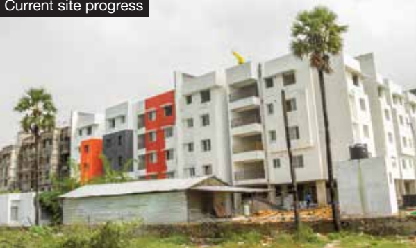
Current site progress
