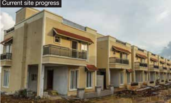
Current site progress
